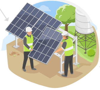
Construction and commissioning
